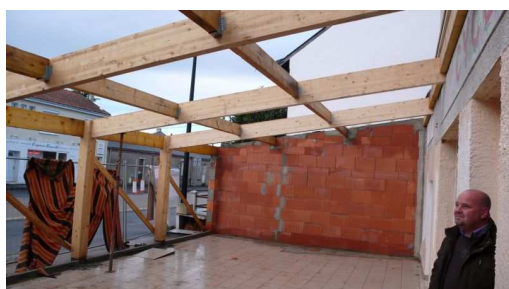
◀ THE ROOF GOES ON
